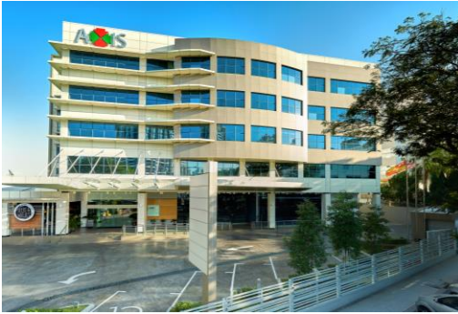
Axis Business Park (Block C)
