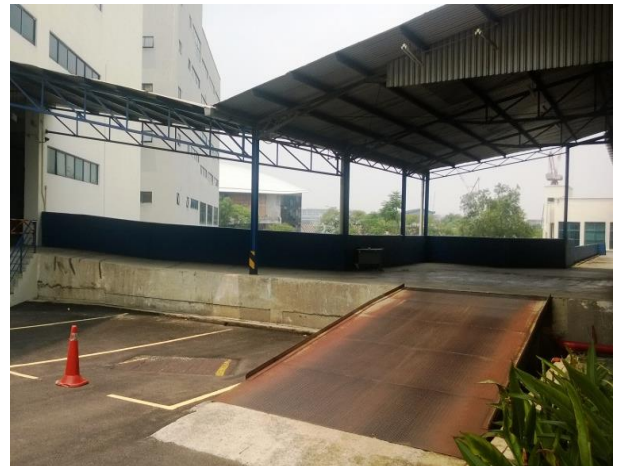
Loading area with 2 loading bays
